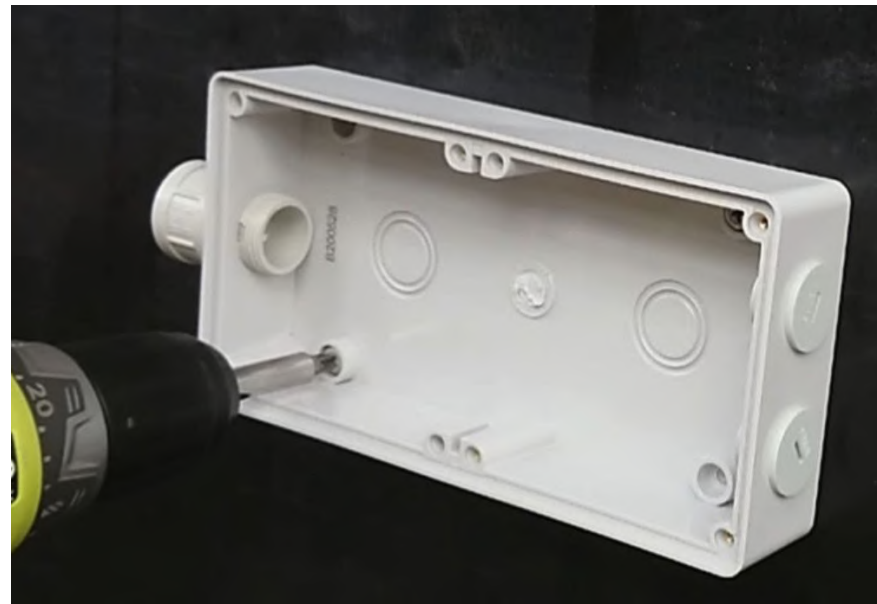
1 - Mount Enclosure Base to Wall
